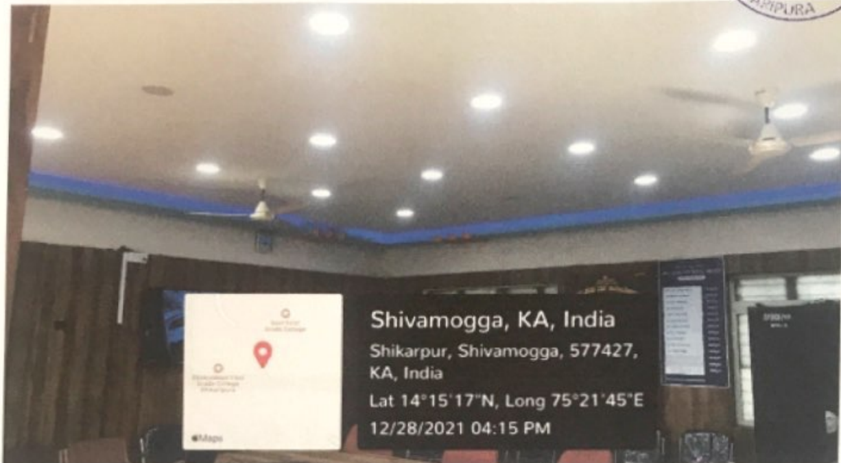
LED BULB FACILITY IN THE PRINCIPAL CHAMBER
