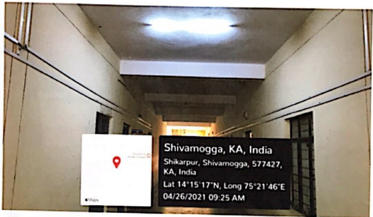
Led bulb facility in the corridor
