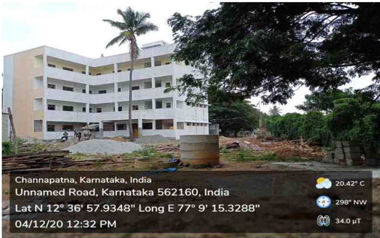
Newly Constructed Building
